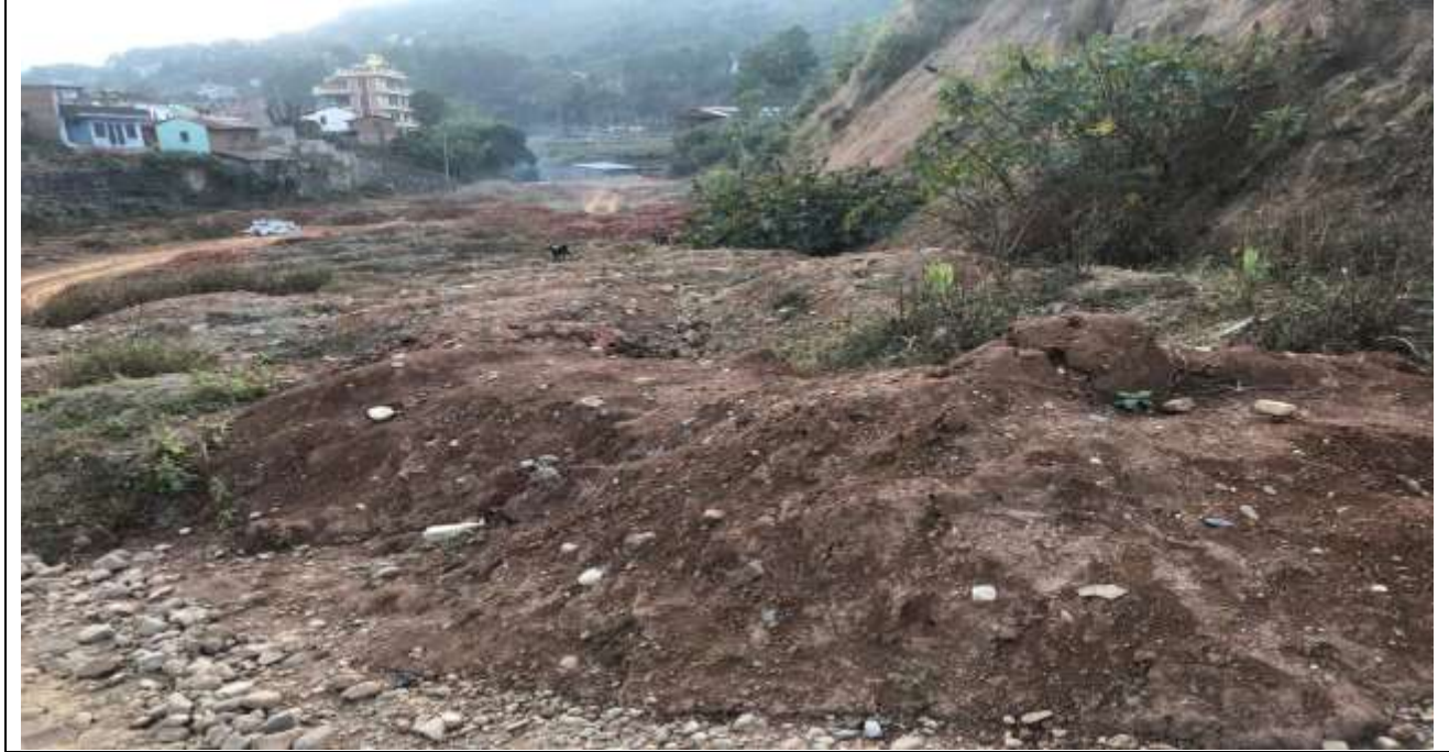
Spoil deposit site Odarechaur Road (20 m away from the chainage 0+000) outer side.
